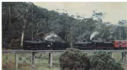
Train on trestle bridge
