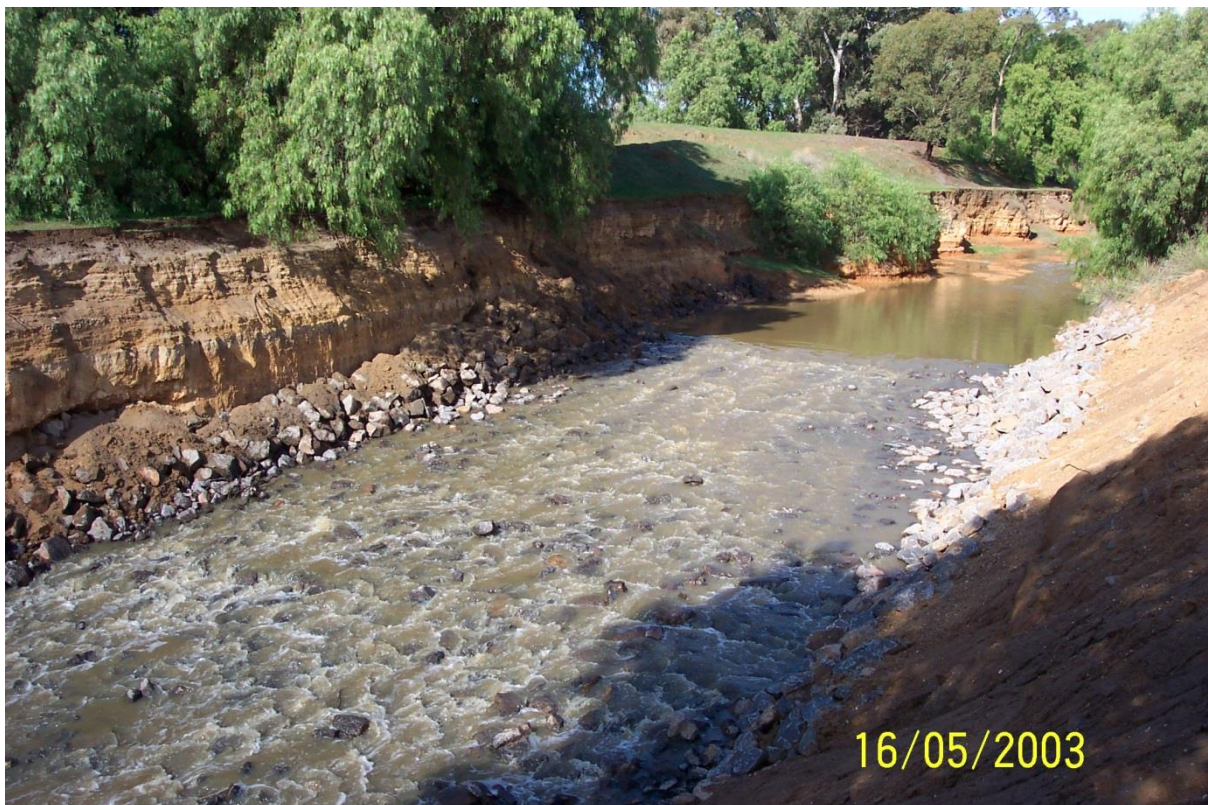
A rock chute is constructed to stabilise the bed and banks to prevent further erosion
