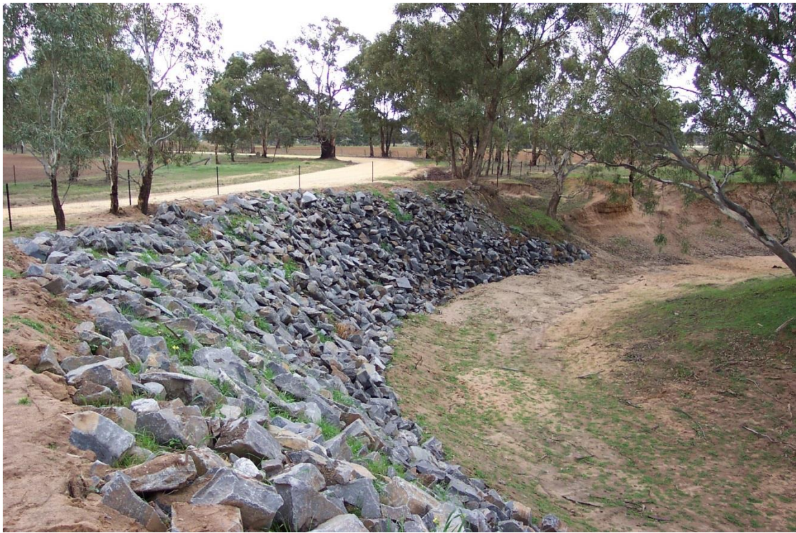
Rock is added to the fast flowing bend of the waterway to prevent further erosion
