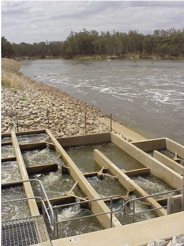
A fish ladder is built in the Murray River Gunbower
