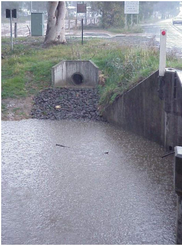
Stormwater outlet from roadside drainage
