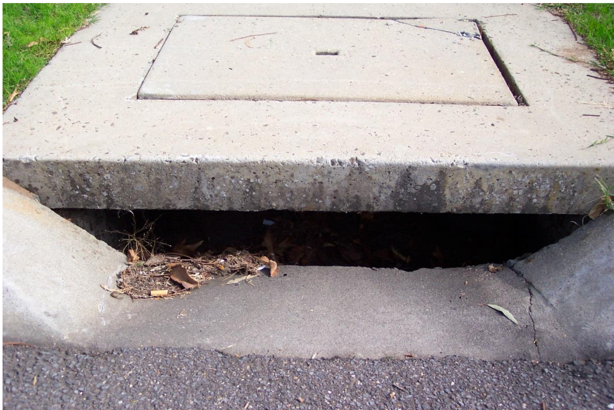
Roadside stormwater pit
