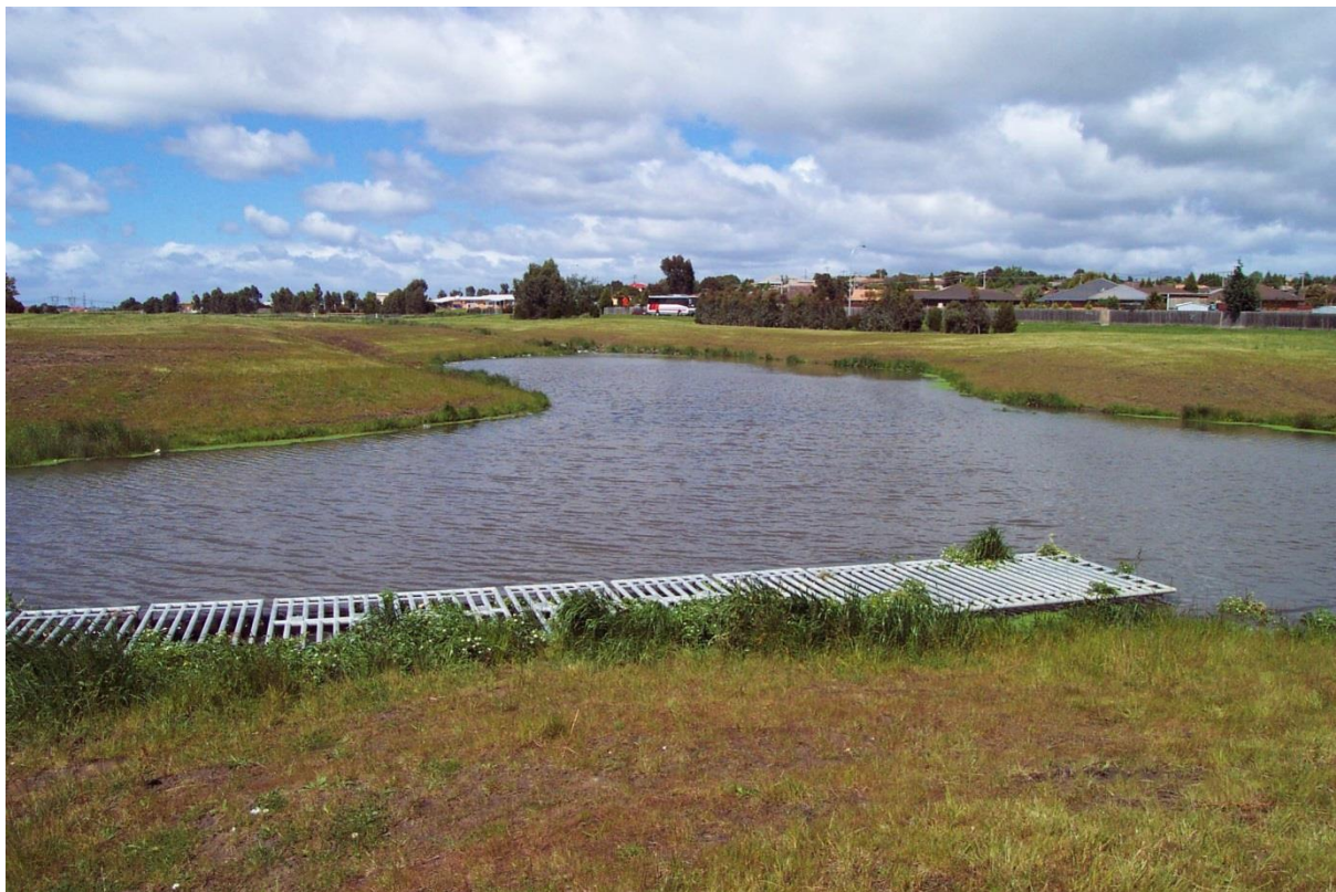
Wetland sediment and litter trap near large housing development
