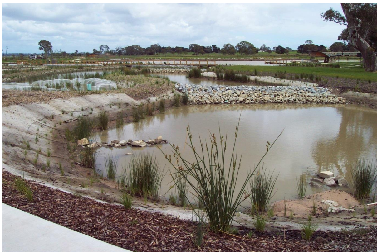
Best practice example of stormwater settling ponds in new housing estates
