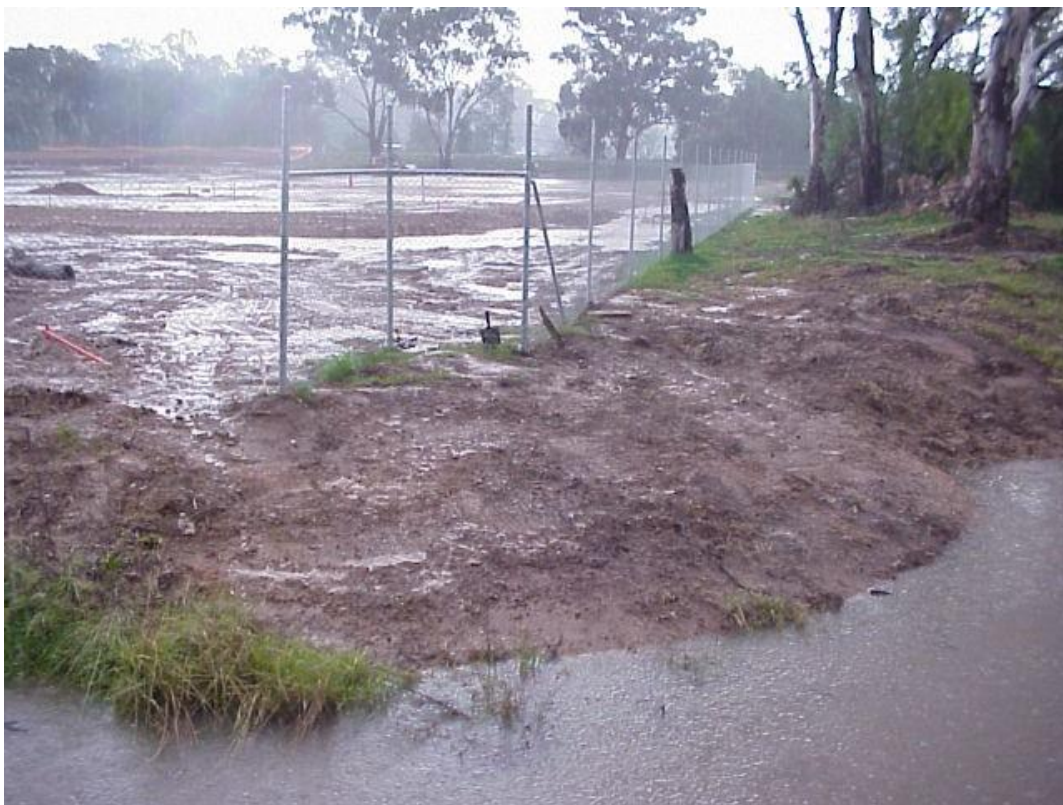
Nothing stopping sediment washing into waterway from building development site
