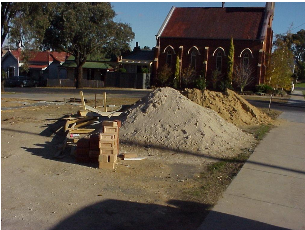
Unsecured sediment on building site in an urban area. Imagine what rainfall will do . . . .
