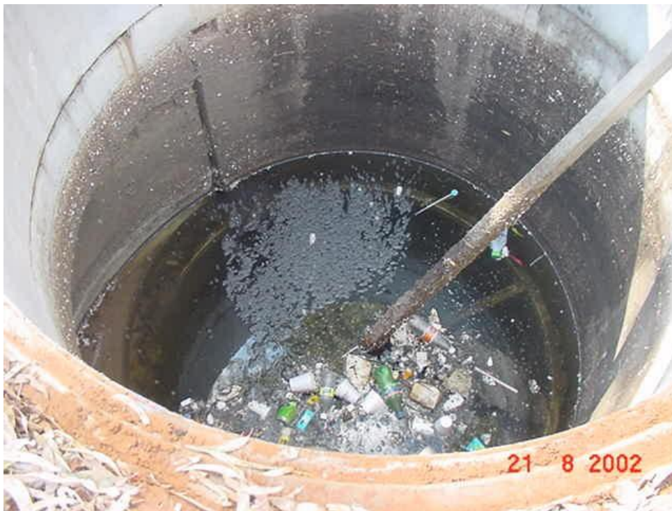
Litter traps catch rubbish before it enters waterways
