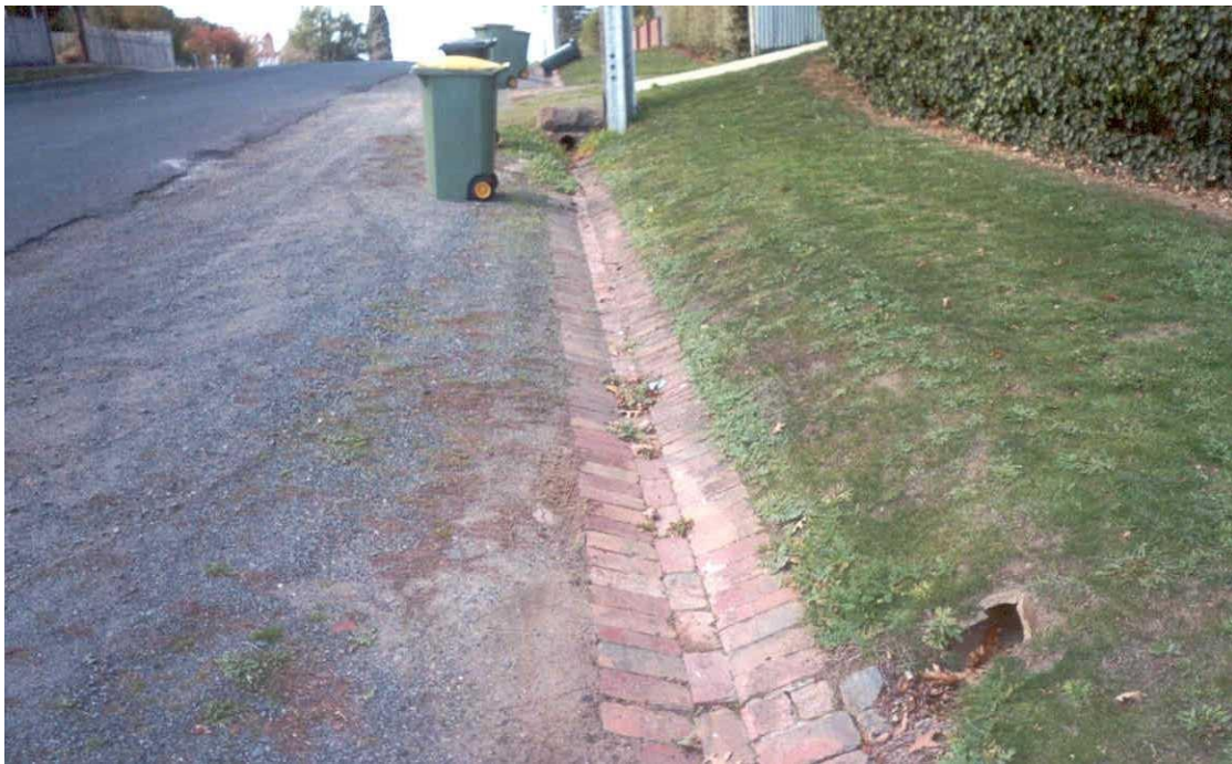
Brick lined drain in suburban area
