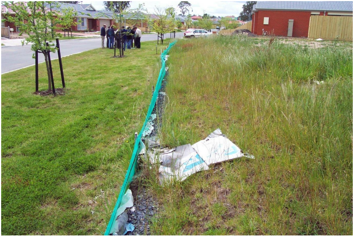
Sediment and litter barrier installed at building site
