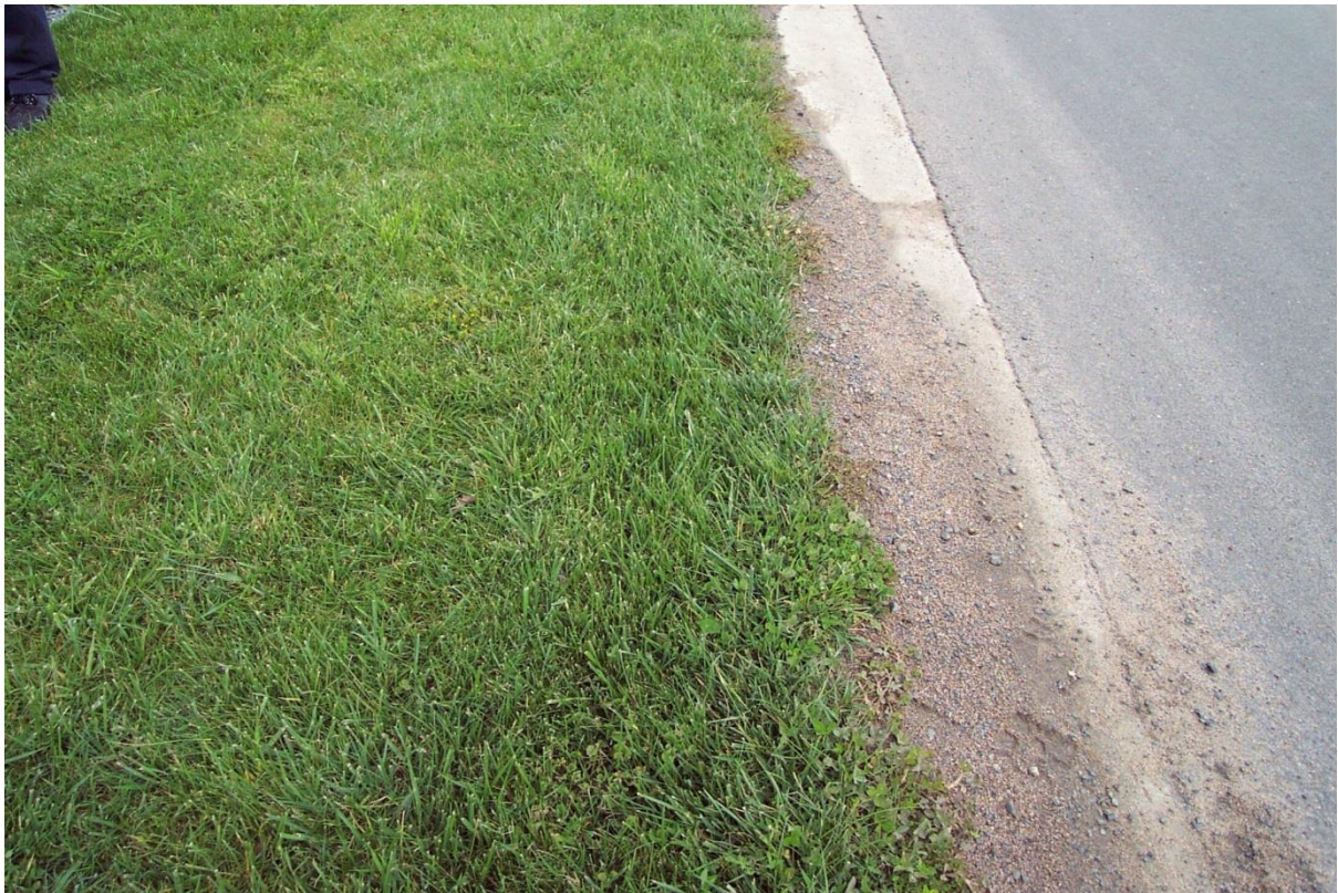
Grassed roadside verges filter sediment and absorb rainfall
