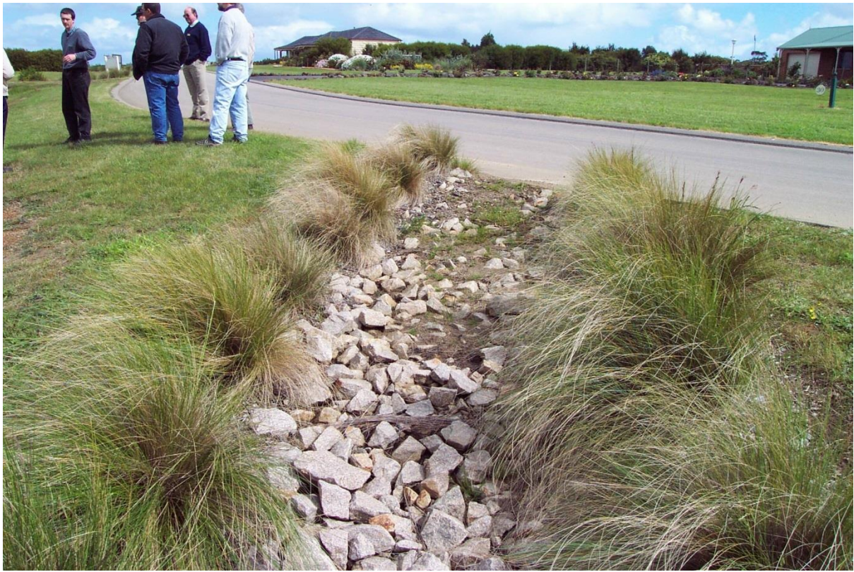
Best practice example of stormwater swathe catching runoff from a suburban roadway
