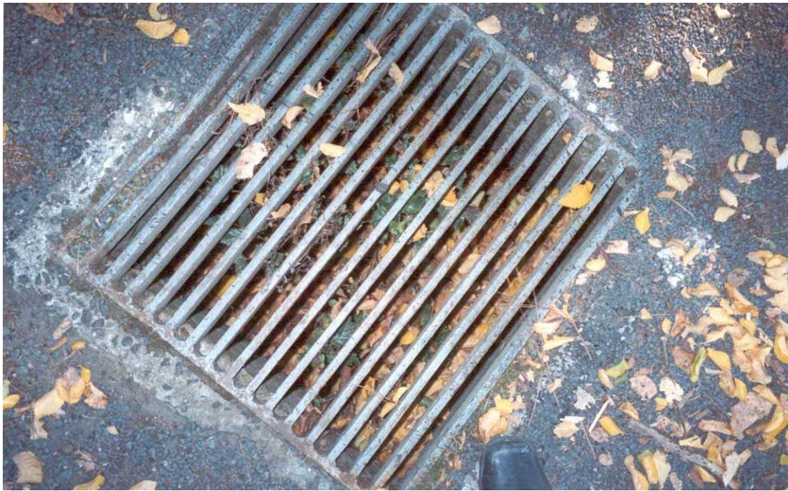
Stormwater pit clogged with autumn leaves
