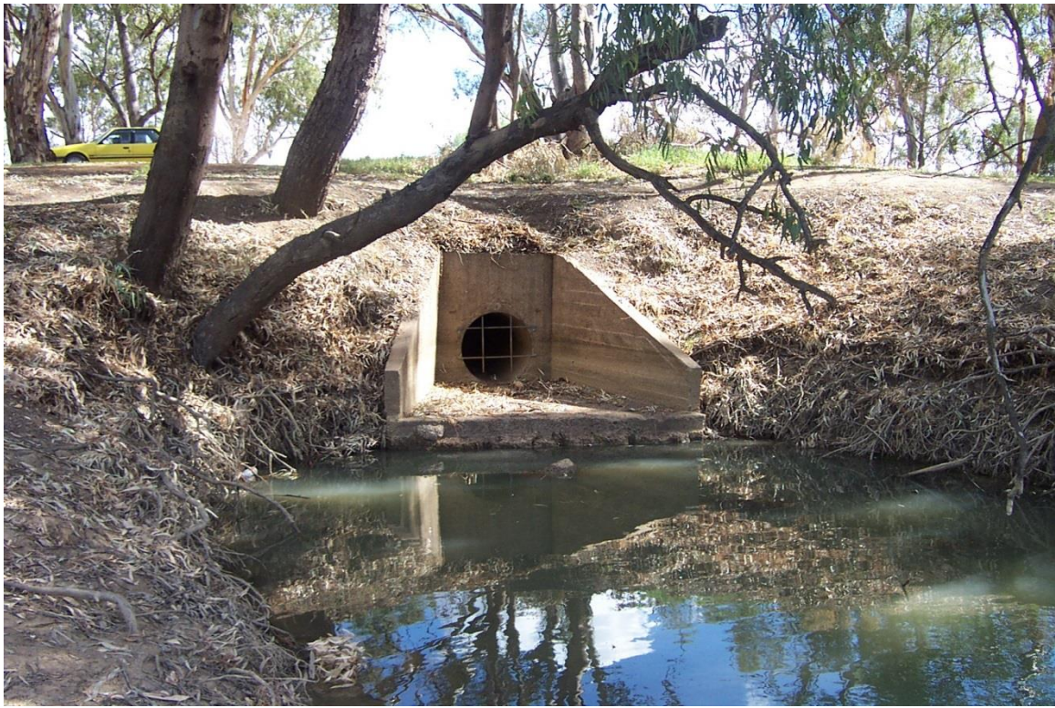
Stormwater outlet from roads into adjacent billabong
