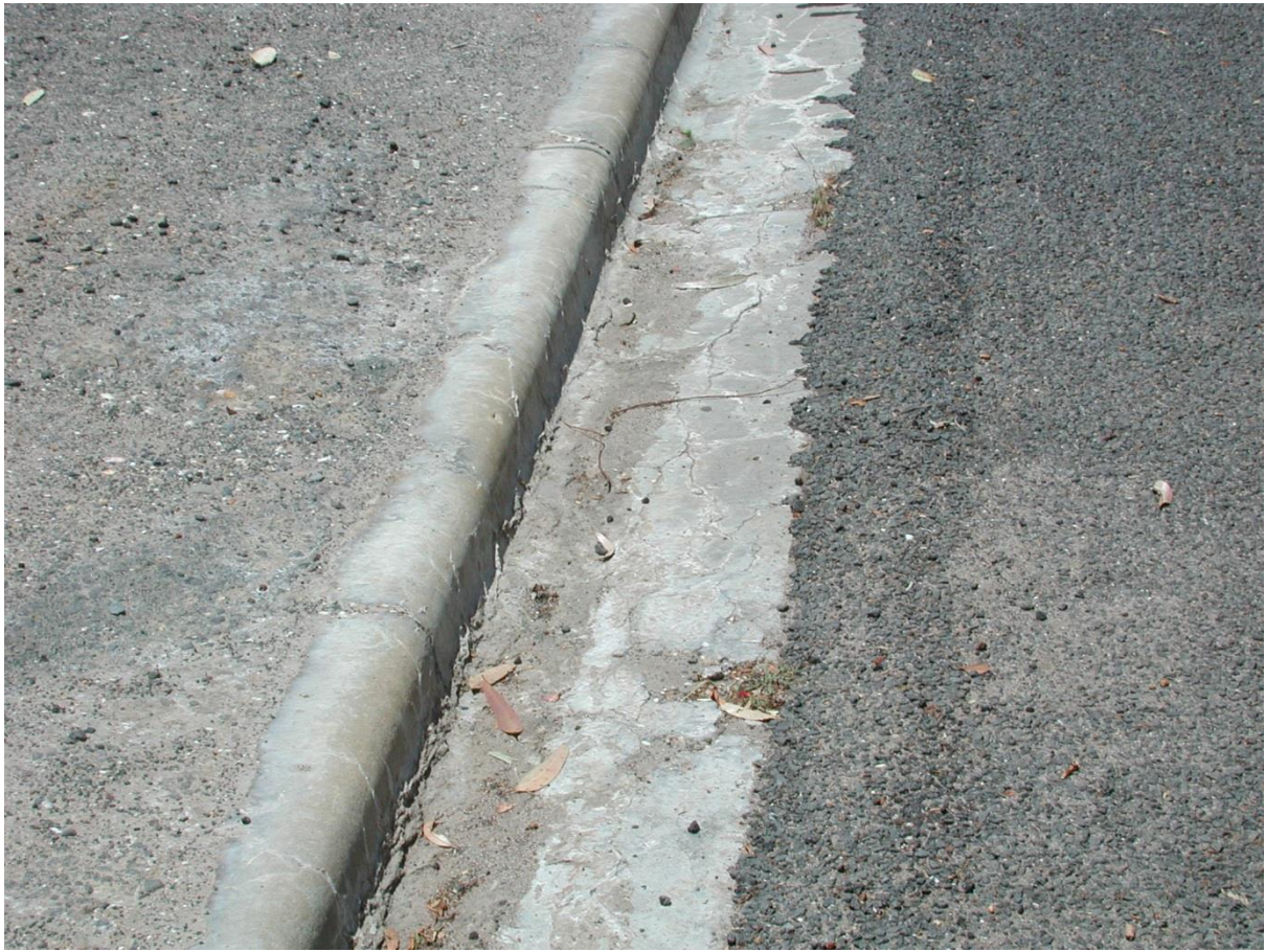
Cracked concrete gutters
