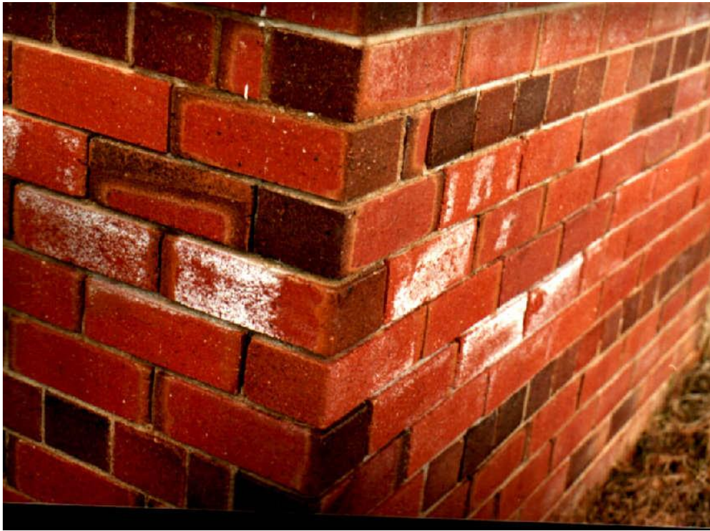
Salt showing on brickwork
