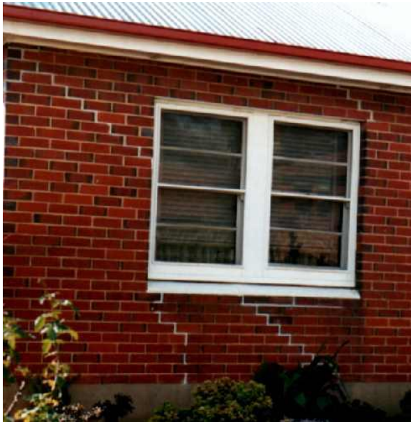
Cracks in a wall caused by salinity
