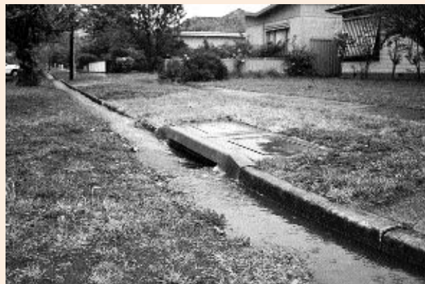
After heavy rain
